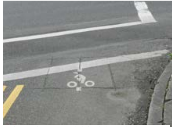
The bicycle detection symbol should be used in bike lanes or shared lanes to depict the "sweet spot" for optimum detection regardless of detection technology.
