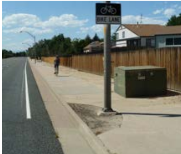
Example of existing bicycle facility with approximately 2-feet of space left of the gutter seam resulting in a condition where there is an 11' travel lane, and 4' bike lane on Smoky Hill Road.
