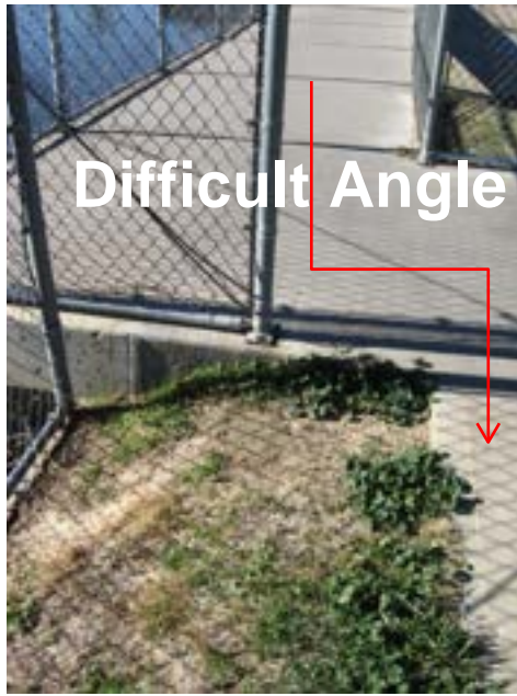
Transition to bridge crossing: Trail widening and railing modifications needed
