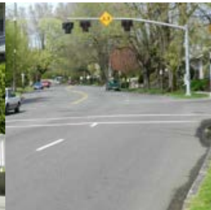
HAWK Signal Across Arterial with Bike/Ped Crossing Warning Sign
