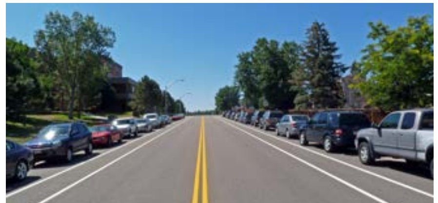
Many of Aurora's streets can be retrofitted to accommodate bicycle facilities. Here vehicle lane widths have been reduced to accommodate bike lanes.
